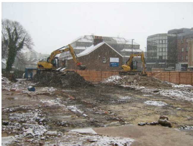
General view of the excavation (in the snow)
